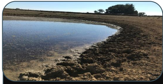
Mechanical damage by livestock
